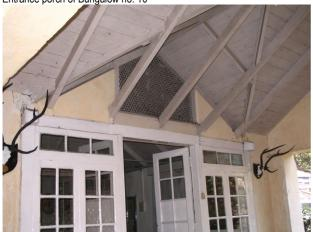
Internal view with sloping roof supported on wooden truss
